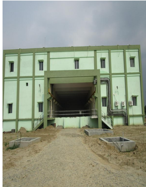
MAIN PUMPING STATION:-
